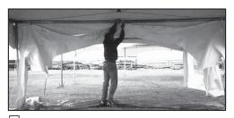
3. Attach clips to Cable: Slide Wall.
